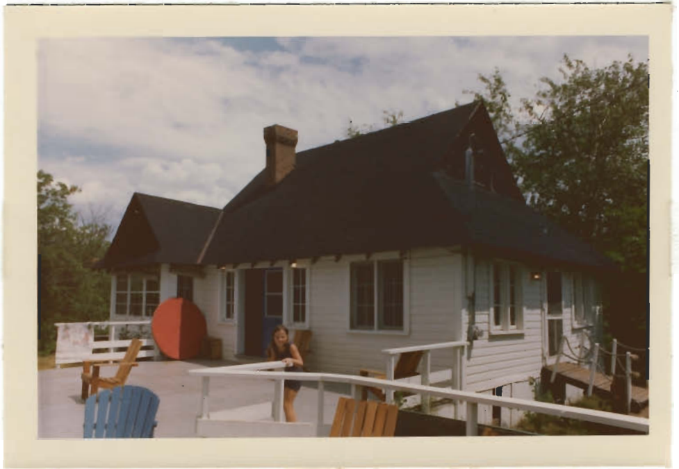
Front of club house from the western corner of the porch.
