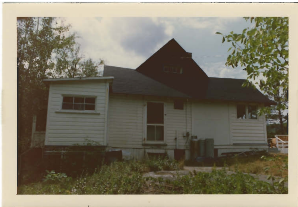
North East side of club house showing rear entrance to kitchen.
